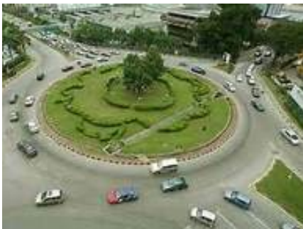
(a) Traffic circle
